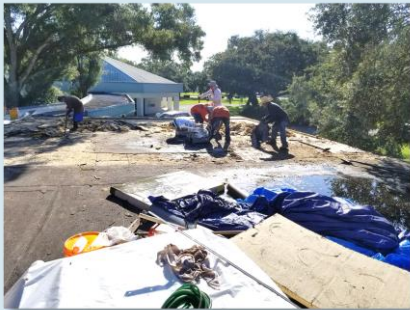
Removing the old roof from over the office
