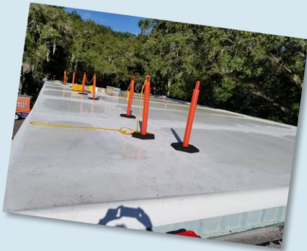
Overview of hall roof looking towards kitchen
