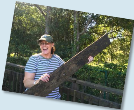
Amy is happy to demolish the rotting deck
