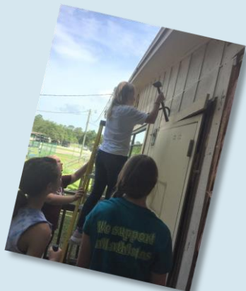
Sydney Removing part of a door jamb
