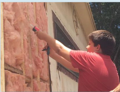
Austin putting in liquid nails on studs
