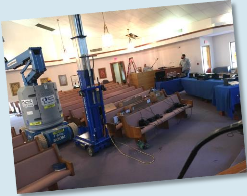
Both lifts in and lights unpacked ready to install
