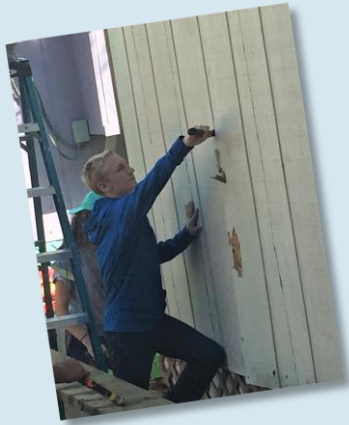
Conner ripping off rotten siding
